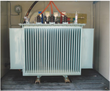
Transformer Chamber
